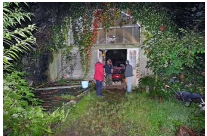
The north entrance to Ho 1
